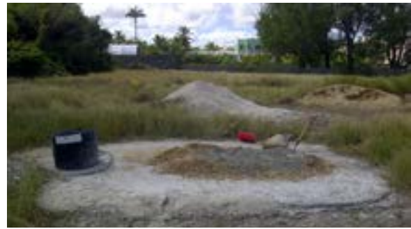
Mixing concrete on a concrete blinding bed
