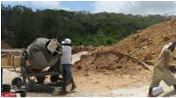
Mixing concrete in a concrete mixer
